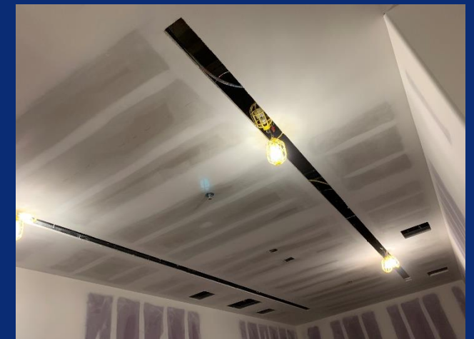
Finishing Drywall Ceilings in Area G
