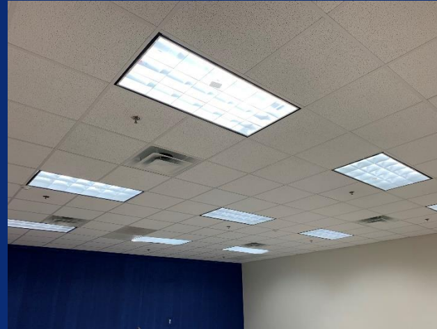
Acoustical Ceiling Tiles in Area K Classroom
