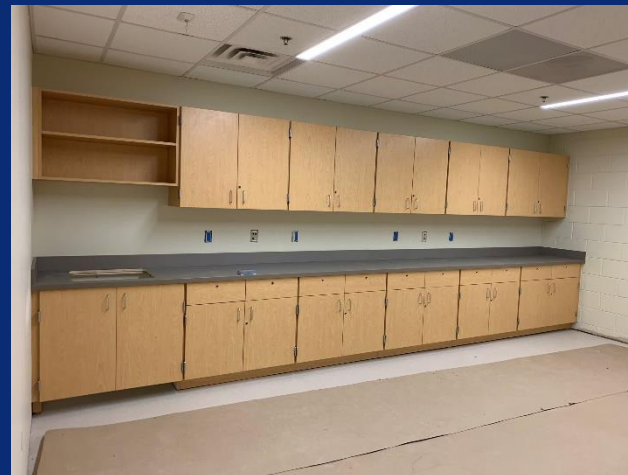
Casework in Area E Teacher Workroom
